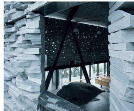
Glued directly to the wall, secured with mechanical fixings, cement-based or elastic joints. Skifer Hotel – Oppdal, Mortensrud kirke - Oppdal.
