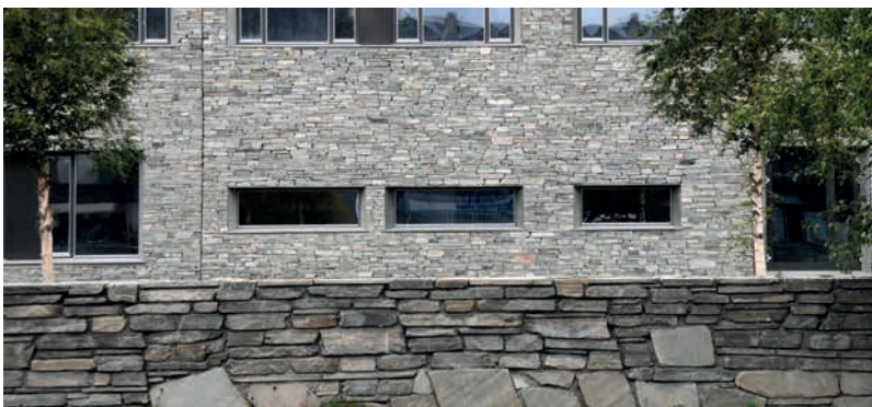
Glued directly to the wall, secured with mechanical fixings, cement-based or elastic joints. Skifer Hotel – Oppdal, Mortensrud kirke - Oppdal.
