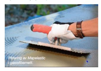
Membrane is applied at a thickness of at least 2 mm, and will protect the underlying structure and reduce the risk of scale deposits on outdoor use.
